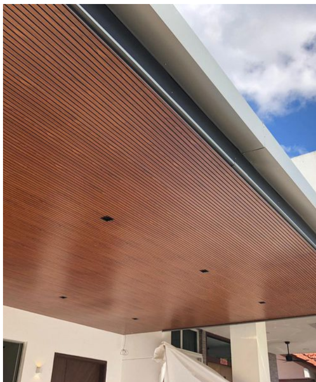
Car Porch Ceiling
